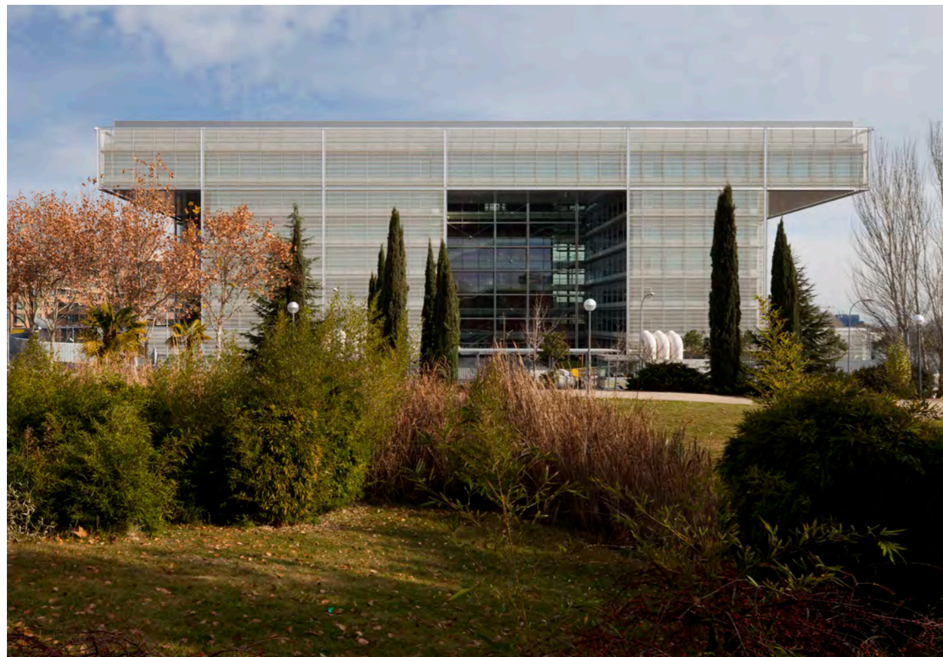
The ceramic coating on the solar reflector tubes in front of the outer façades catches the light and diffuses it into the building at a dimmed level.
