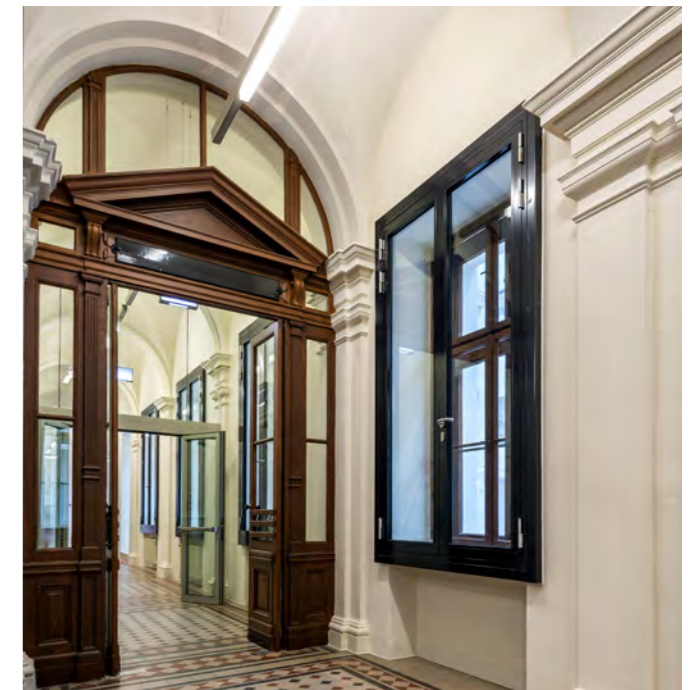
For the windows and doors, the heat-insulated system Janisol HI was installed at the new university campus. Janisol C4 EI60 and Janisol 2 EI30 fire-proof doors were also installed.
