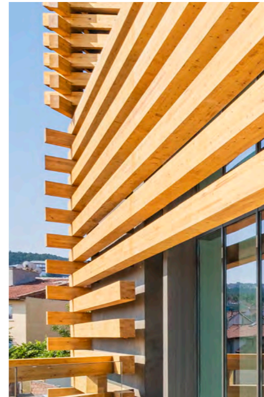
The mounted façades made from squared-edge timber are an homage to the centuries-old tradition of woodwork in the region. They have the added benefit of providing sun protection where the glass façades are.
