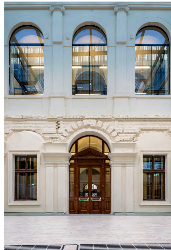
A transparent atrium – constructed from the Jansen VISS façade steel profile system – connects the library to the main university building, making it one continuous space.
