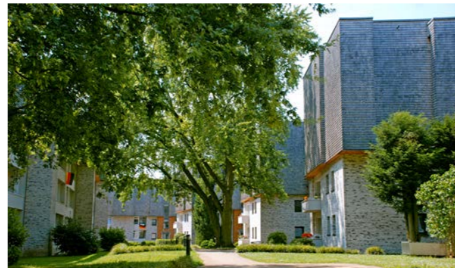
Densification through upwards expansion. Upwards expansion allows the large areas of trees and shrubs to be retained. The spatial proportions and shading of the free spaces change (Bebelallee housing development, Hamburg, Germany).
