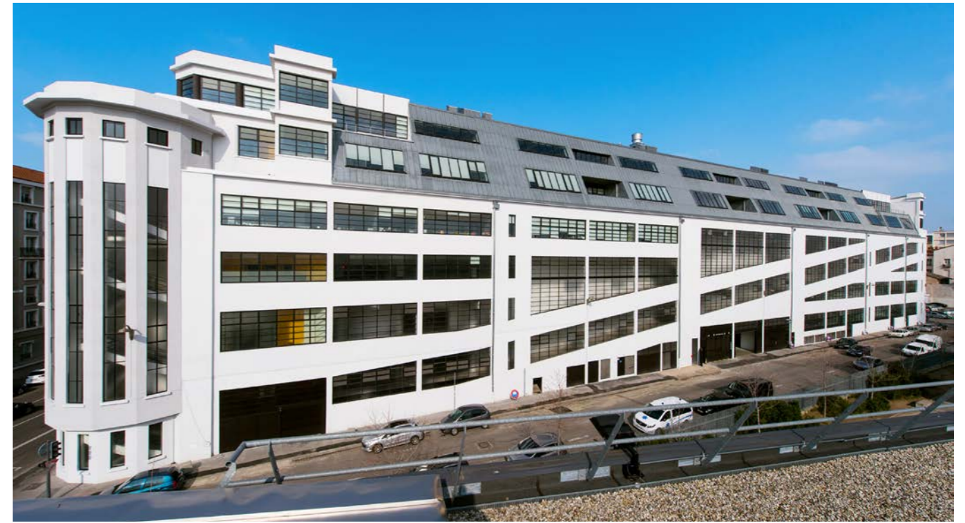
The internal ramps can be clearly seen in the façade on Rue Béchevelin. The small window and fixed glazing sections were reconstructed using Janisol Arte so that they remained true to the original.
