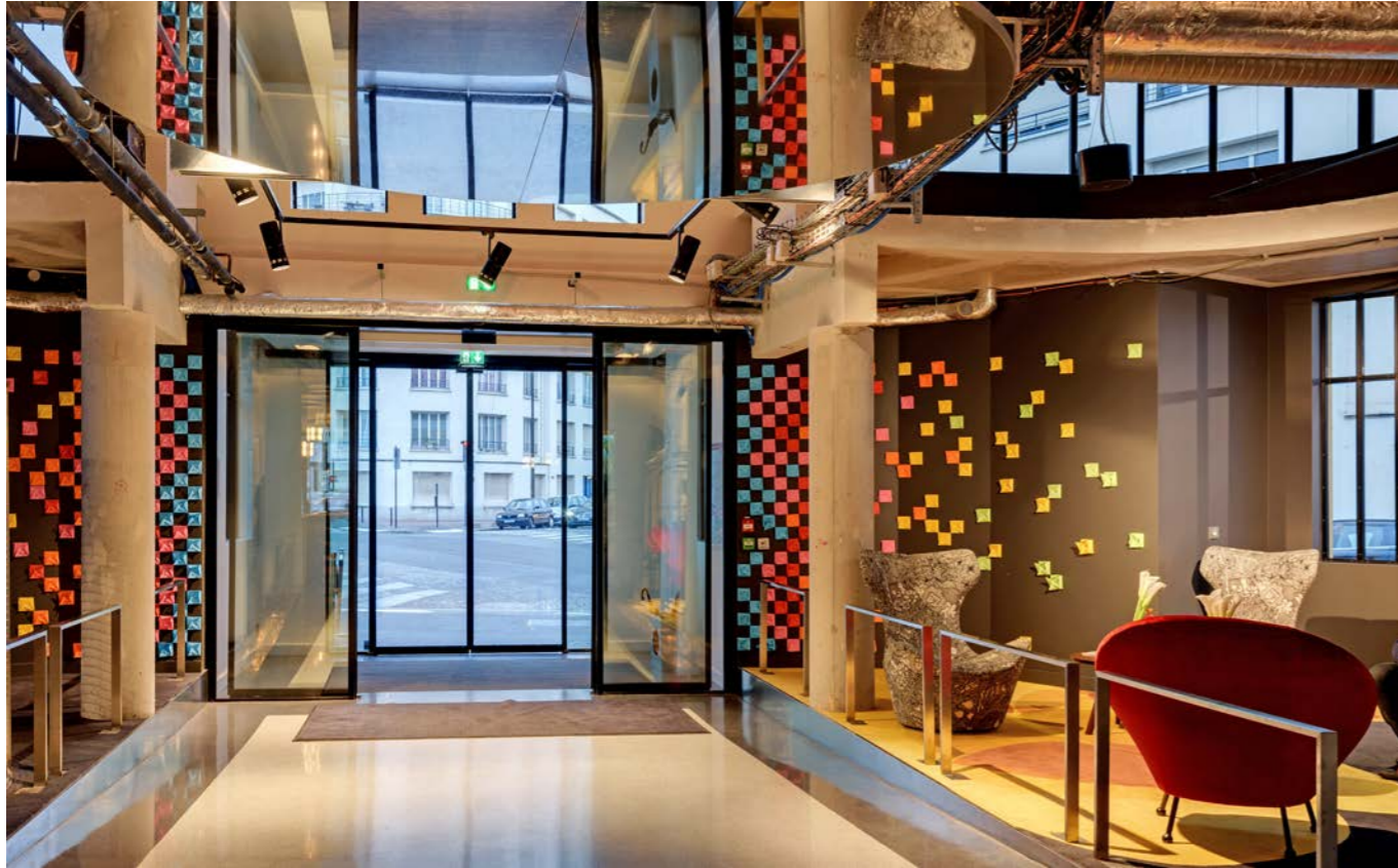
Glass sliding doors with slimline frames made from Janisol Arte steel profile systems underline the high aesthetic requirements placed on the design.
