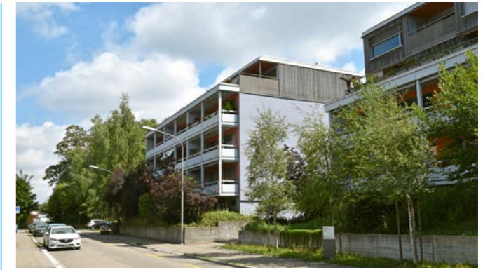
Densification through upwards expansion and renovation of the existing building in order to retain unique structural features (Irchel retirement homes, Zürich, Switzerland).
