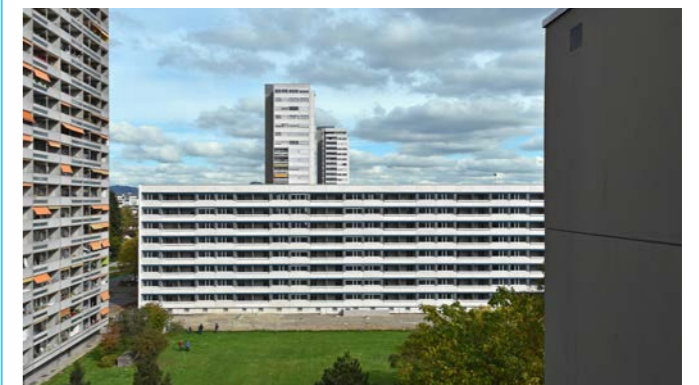
Renovation and supplementation of the existing building with spatial layering to extend the living space in close cooperation with the heritage preservation authorities (Tscharnergut housing development, Bern, Switzerland).
