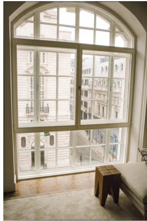
The architects opted to update the large window areas in keeping with the old style using steel profile systems.
