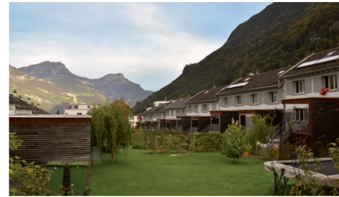
Densification through supplementing with spatial layering, renovation of existing buildings and structuring of free spaces (Turmatt workers' housing development, Altdorf, Switzerland).
